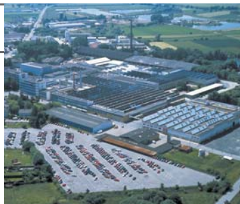
Stiebel Eltron's plant in Holzminden, Germany.
